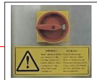
MAINS SUPPLY ISOLATOR
